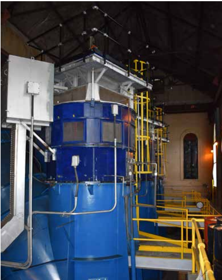
P27. Interior of Hydroelectric Plant, in 1983 (top) and 2017 (bottom). (Resource 36)
