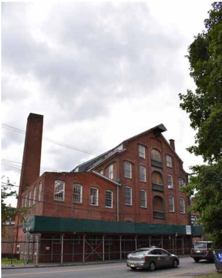
P18. Rogers Locomotive Company Erecting Shop, in 1971 (top) and 2017 (bottom). (Resource 15)
