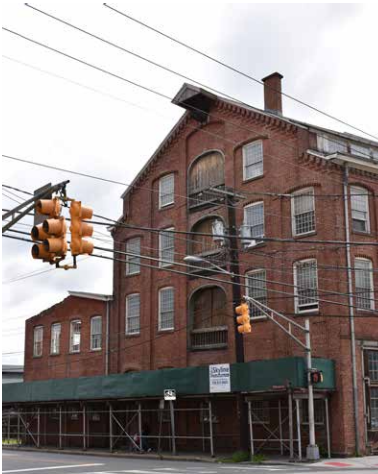
P15. Rogers Locomotive Company Erecting Shop, in 1971 (top) and 2017 (bottom). (Resource 15)
