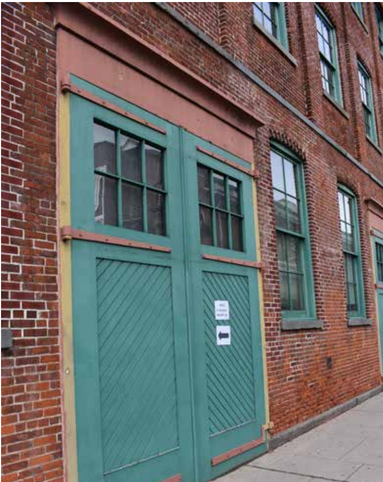
P6. Rogers Locomotive Company Frame Fitting Shop and Administrative Building, in 1971 (top) and 2017 (bottom). (Resource 05)
