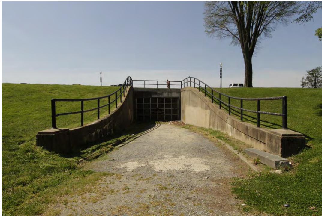
Fig. 94: View to the southwest of the underground entrance to the Parkway Drive NW storage room. (Torkelson 2021)
