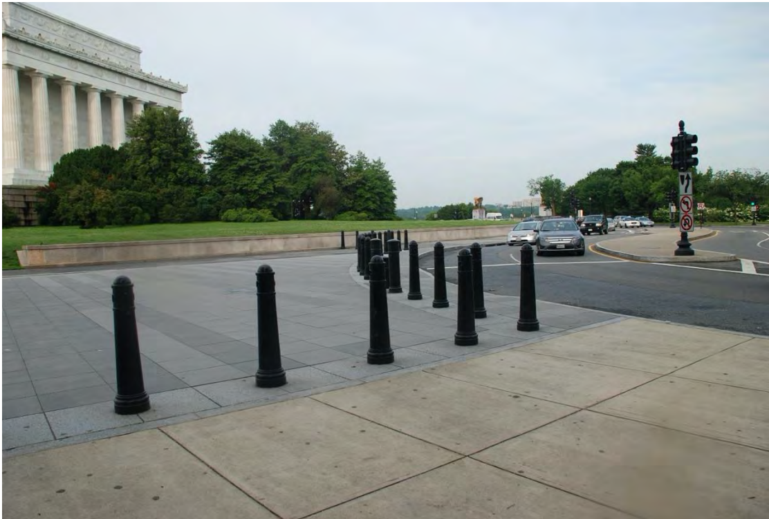
Fig. 43: Security bollards were installed in 2008 as part of a larger restoration and rehabilitation project for the Lincoln Memorial structure and landscape. (Lowe 2012a)
