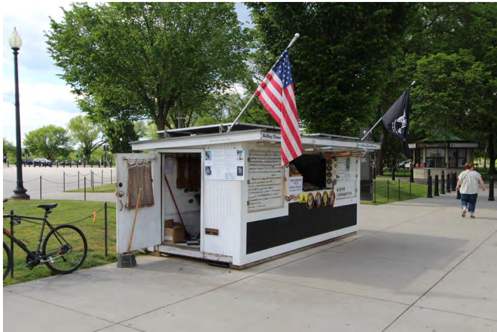
Fig. 95: View to the northwest of the non-contributing (incompatible) POW/MIA structure (aka the Last Firebase). (Torkelson 2021)
