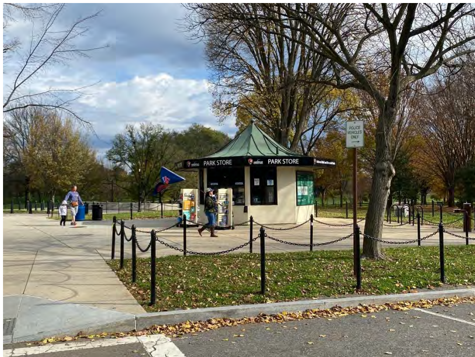
Fig. 85: View to the north of the non-contributing park store and information kiosk adjacent to the Korean War Veterans Memorial. (Mason 2021)
