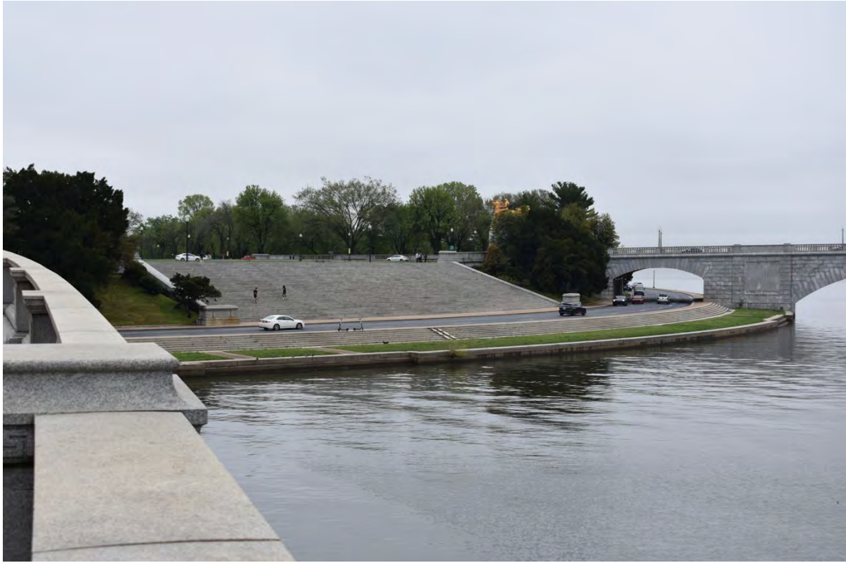
Fig. 55: View to the southeast of the Watergate Steps area's steep topography, sloping down to the Potomac River. Note the Watergate Steps and the surrounding steeply sloped planting beds and retaining walls. (Lester 2021)
