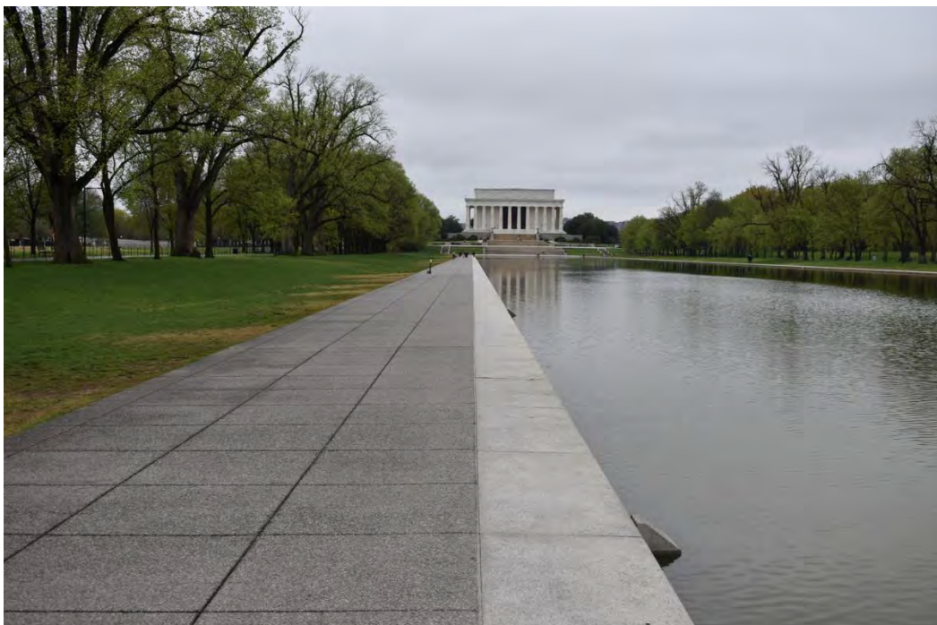
Fig. 79: View to the west showing the historic Reflecting Pool coping and non-contributing walks added by Sasaki in 2010. (Lester 2021)
