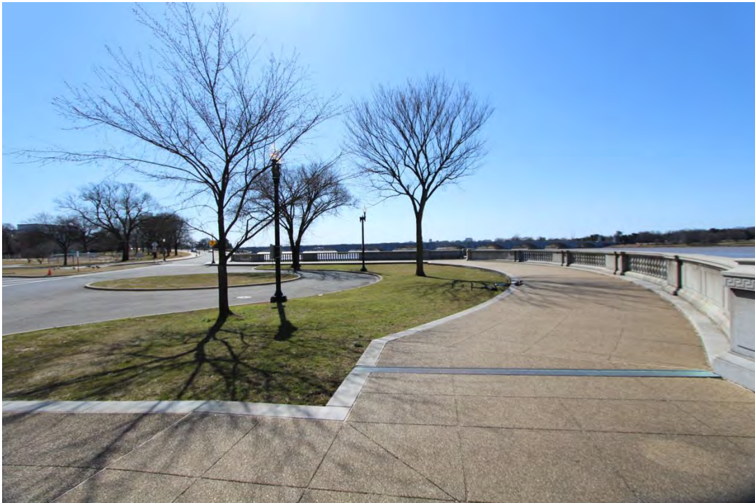
Fig. 74: View to the south showing the historic Belvedere, at the western terminus of Constitution Avenue. Note the traffic circle, granite curbing, and exposed aggregate paving. (Torkelson 2021)
