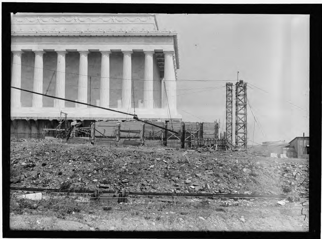
Fig. 27: Lincoln Memorial structure under construction, 1916. (Harris & Ewing Collection, Library of Congress)
