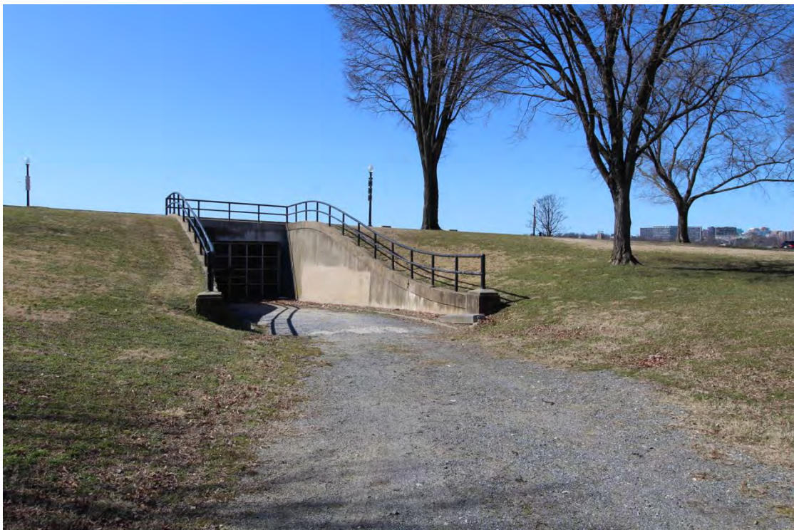
Fig. 75: View to the southwest showing the historic gravel road leading to the storage area under Parkway Drive. (Torkelson 2021)
