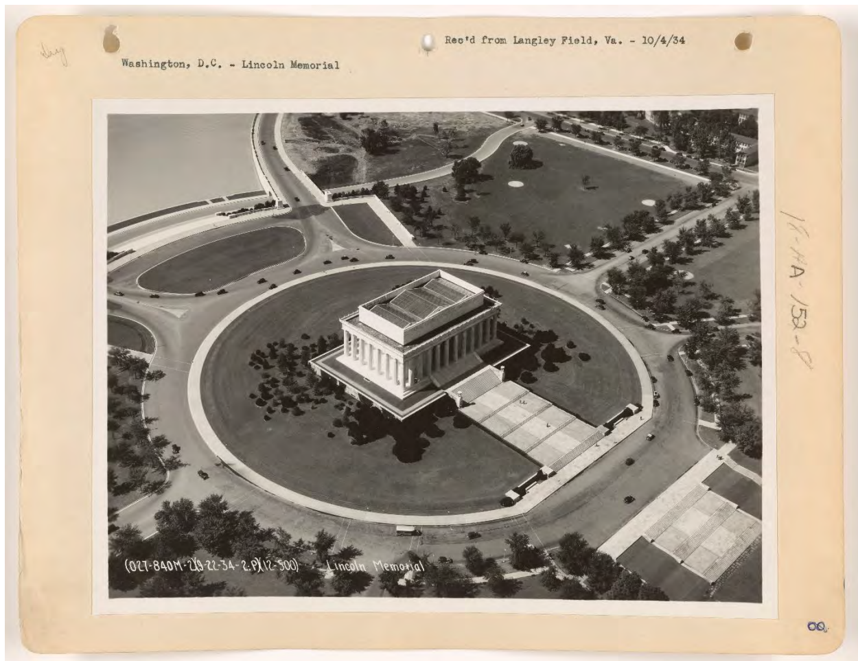
Fig. 33: 1934 view of the site. The storage tunnel is in place northeast of the Watergate Steps. (War Department, Army Air Forces 1934b)
