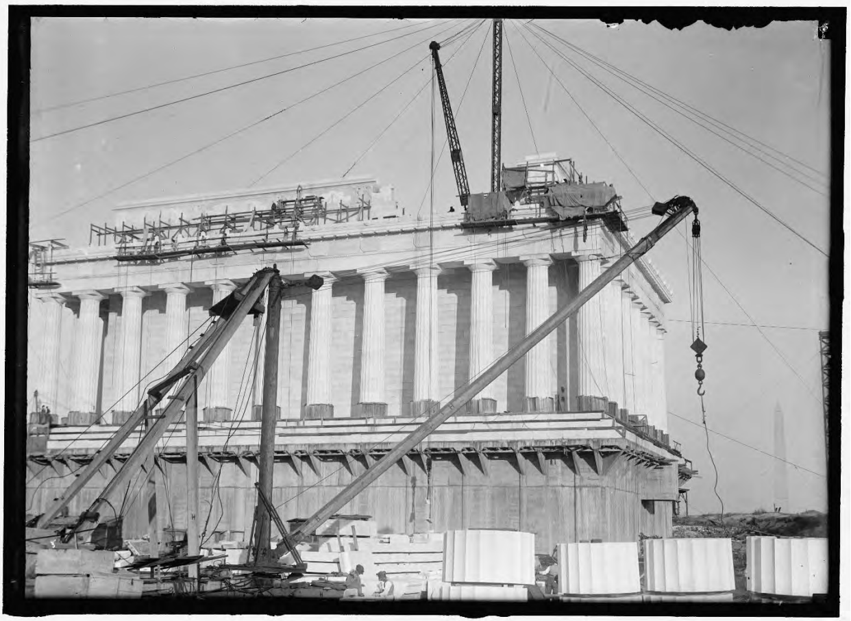
Fig. 26: Lincoln Memorial structure under construction, c. 1916. (Harris & Ewing Collection, Library of Congress)
