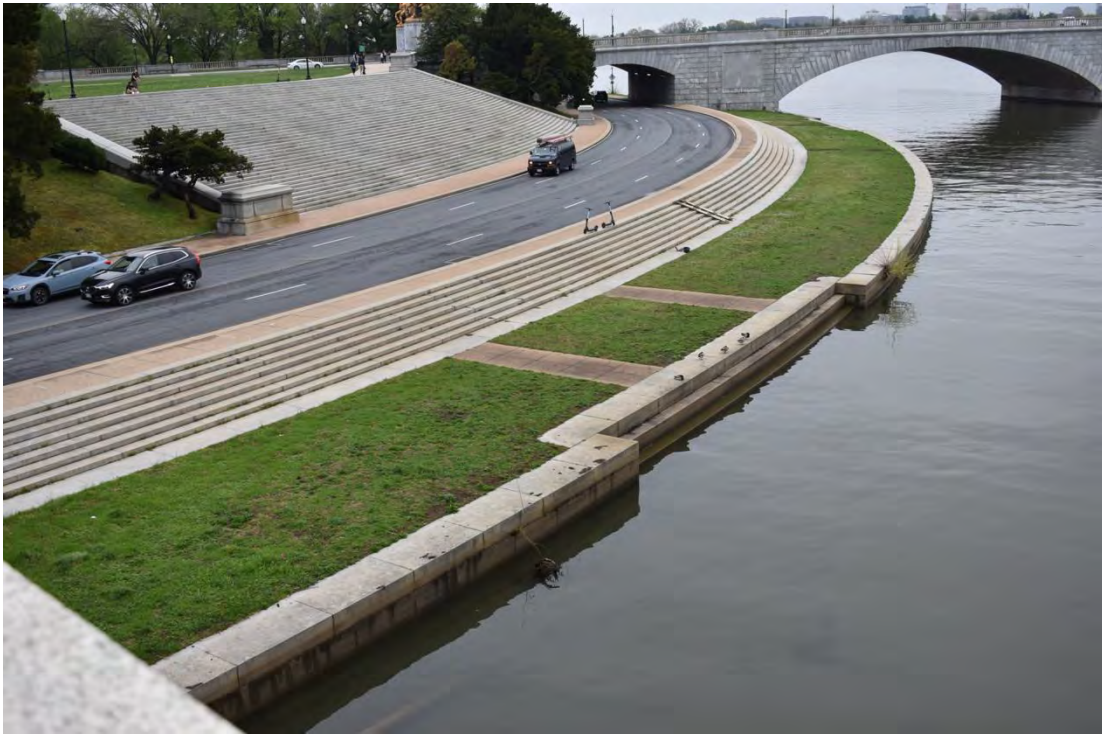
Fig. 80: View to the southeast showing the historic Watergate Steps and associated circulation features. These include the upper and lower steps, Ohio Drive SW, the overpasses, and the various sidewalks. (Lester 2021)
