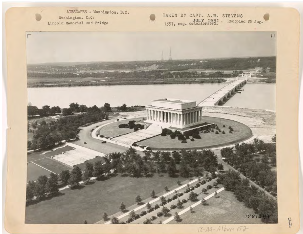
Fig. 56: View to the southwest showing the completed plantings east of the Lincoln Memorial as of 1931. (War Department, Army Air Forces 1931)
