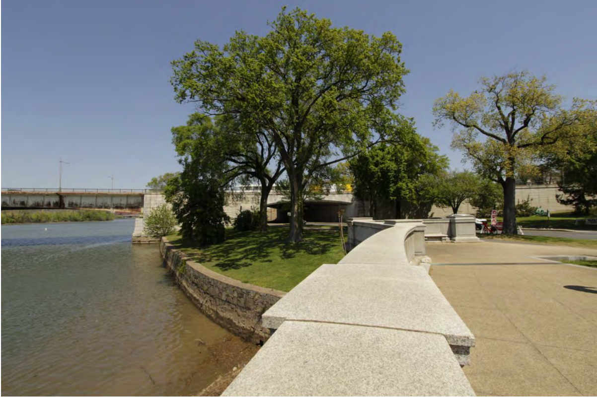
Fig. 52: An example of the topographic edge conditions of the cultural landscape (seen here at the Belvedere), featuring a slight slope terminated by seawalls or other retaining walls. View to the north along Parkway Drive SW of the Theodore Roosevelt Bridge overpass (background). (Torkelson 2021)
