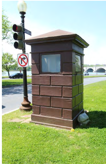
Fig. 92: View to the west of the non-contributing (compatible) guard stand at the corner of Ohio Drive SW and 23rd Street SW. (Torkelson 2021)
