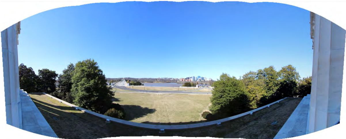
Fig. 98: Panoramic view to the west from the Lincoln Memorial showing the designed fan-shaped viewshed. Note the encroaching mature vegetation at the northwest and southwest corners of the monument that restrict historic views of Parkway Drive NW and the Potomac River. (Torkelson 2021)
