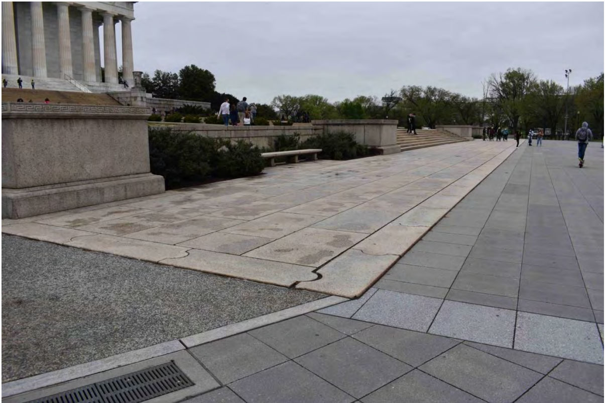
Fig. 71: View to the northwest showing the contributing granite block paving and non-contributing (compatible) modern block paving denoting the former route of Lincoln Memorial Circle. (Lester 2020)
