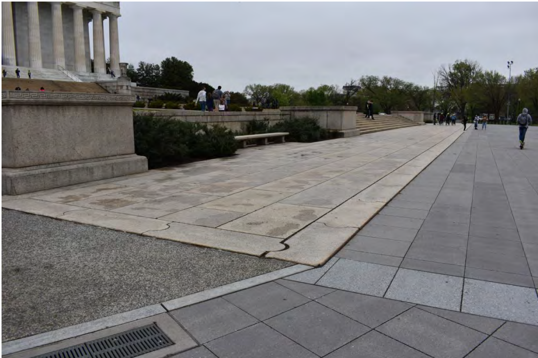
Fig. 78: View to the northeast showing the historic granite paving that marked the edge of the Approachway and Lincoln Memorial Circle. The darker paving of the plaza is non-contributing, as it was added circa 2008. (Lester 2021)
