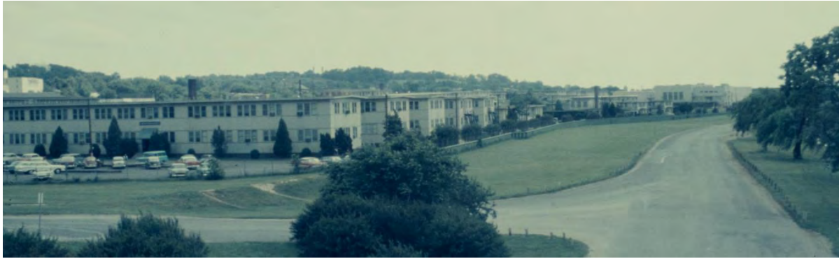
FIGURE 75: Section C features a corrugated metal flood barrier along Anacostia Drive, surrounding the NRS, shown here in 1961. (Excerpt from PR0543A, Emil A. Press slide collection, Historical Society of Washington, D.C.)
