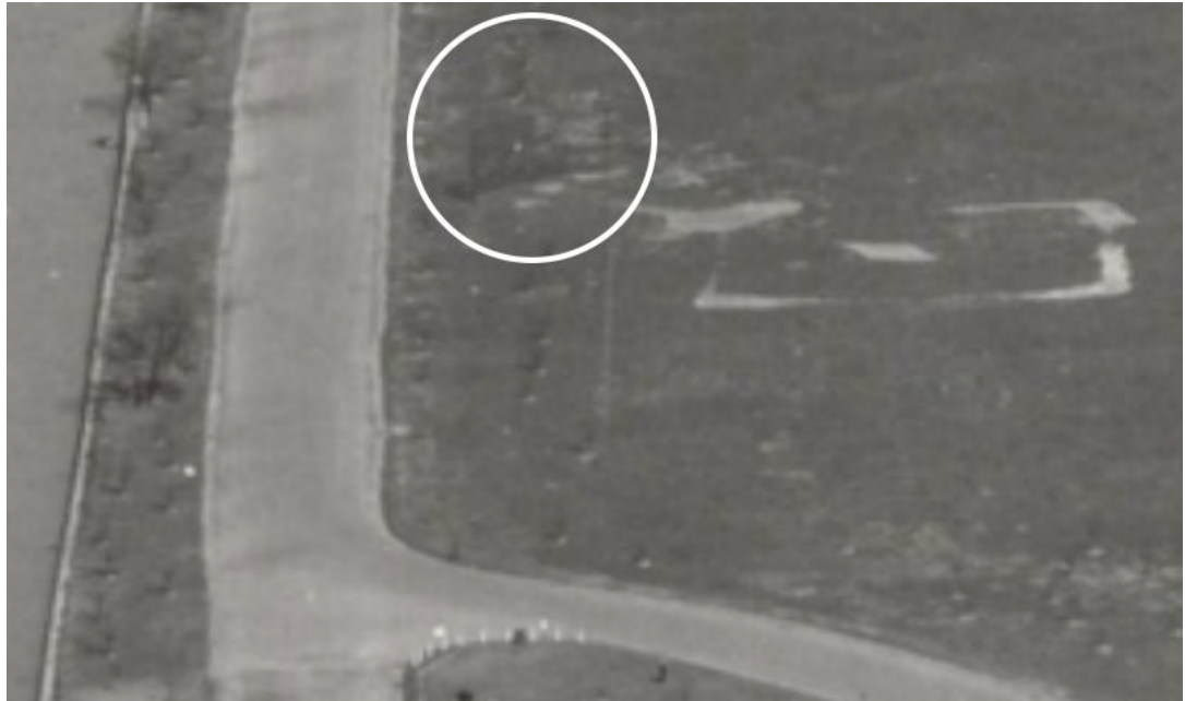
FIGURE 88: The earliest known baseball/softball backstop within the study area, circled in white, was located along Anacostia Drive in Section D, just north of the 11 th Street SE bridge. (Excerpt from RG-18-AA-146-29 National Archives 1933)
