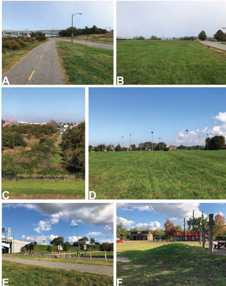
FIGURE 60a-f: Examples of existing topography in Anacostia Park: A) View to the north of steeply sloped topography from the low-lying areas at Anacostia Drive and Good Hope Road SE up to 11th Street SE; B) View to the west of generally flat topography in Section C along Good Hope Road SE; C) View to the north from the WMATA Anacostia park-and-ride of an extant portion of a WPA-era earthen levee; D) View to the north of generally flat topography in Section D; E) View to the northeast of the steeply sloping topography on the south side of the Pennsylvania Avenue SE interchange; F) View to the east of Bicentennial-era berms at the Section D park node (Photos by CLI author 2019-2020).
