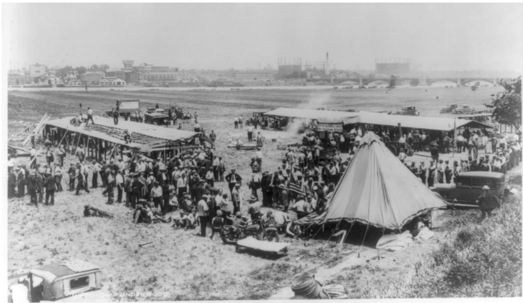
FIGURE 35: The earliest Bonus Army structures built in Section C of the cultural landscape were located on the southern end of the cultural landscape, adjacent to the existing tree nurseries and a small rise near the adjoining neighborhoods that residents used as a dump. The first structure, a bunkhouse located at the right side of the photo, was built with lumber and tar-paper provided by Police Chief Glassford. Using found materials, veterans continued to expand the camp. (Underwood and Underwood, Library of Congress Prints and Photographs Division, Washington, D.C., 1932a)
