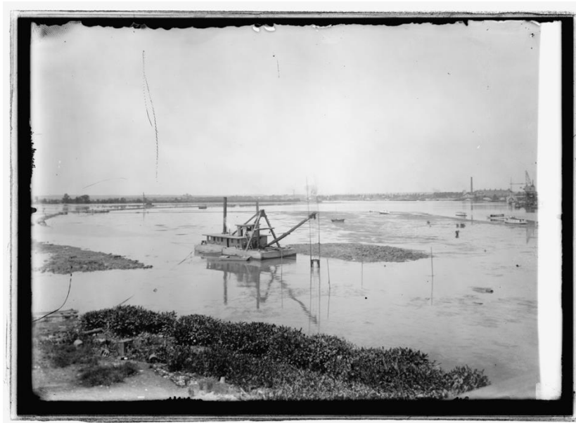
FIGURE 18: Dredge boats like this one were used to reclaim land from the Anacostia River in order to create Anacostia Park. View to the west, 1912. The Washington Navy Yard is pictured at right. (National Photo Company Collection, Library of Congress)
