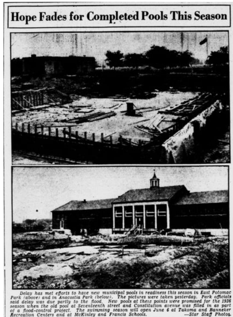
FIGURE 42: Construction of the Anacostia Pool began in 1935, and was completed in 1937 using PWA funding. A flood in 1936 delayed construction and required new reinforced concrete piles. ( Evening Star , May 15, 1936: A3)
