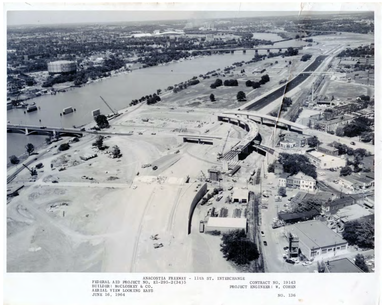
FIGURE 53: View to the northeast from Section C with the 11 th Street SE bridge at left. This 1964 photograph shows the significant changes made to the cultural landscape in Sections C and D caused by construction of the Anacostia Freeway. (Stewart Brothers, “Anacostia Freeway – 11 th Street Interchange,” District Department of Transportation Historic Collections)
