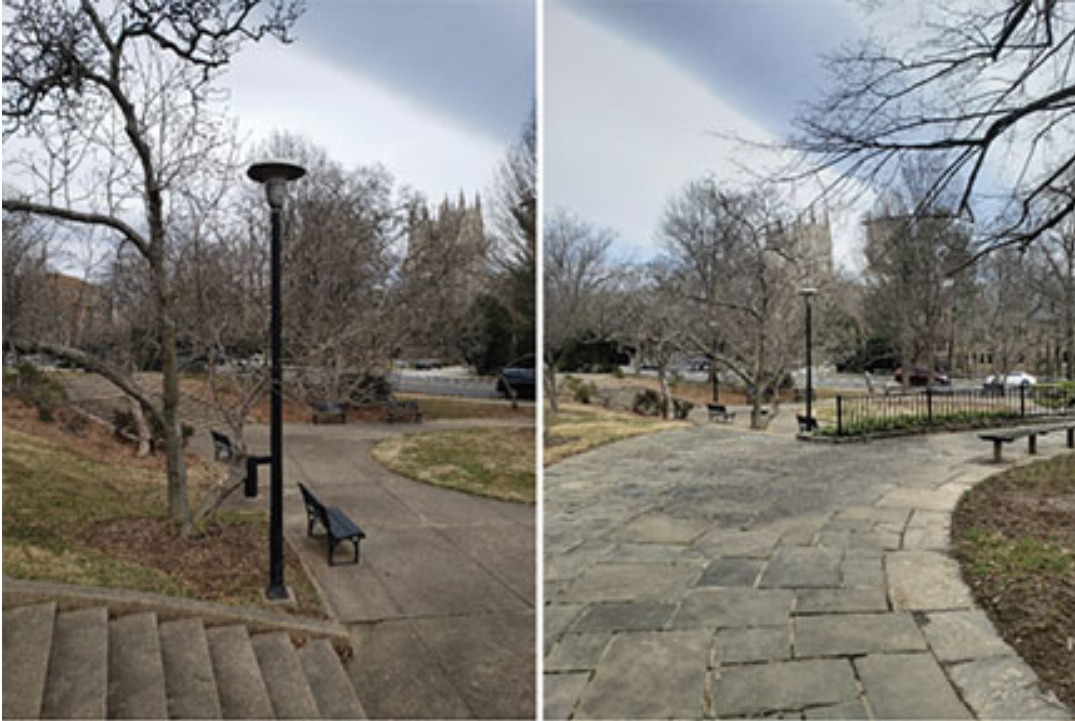
Typical circulation conditions at the Bryce Park cultural landscape include scored-concrete walkways and staircases on the northwest, central, and southeast terraces (left) and Pennsylvania bluestone paving on the southwest terrace (right). (Photos by the CLI author, March 2019)
