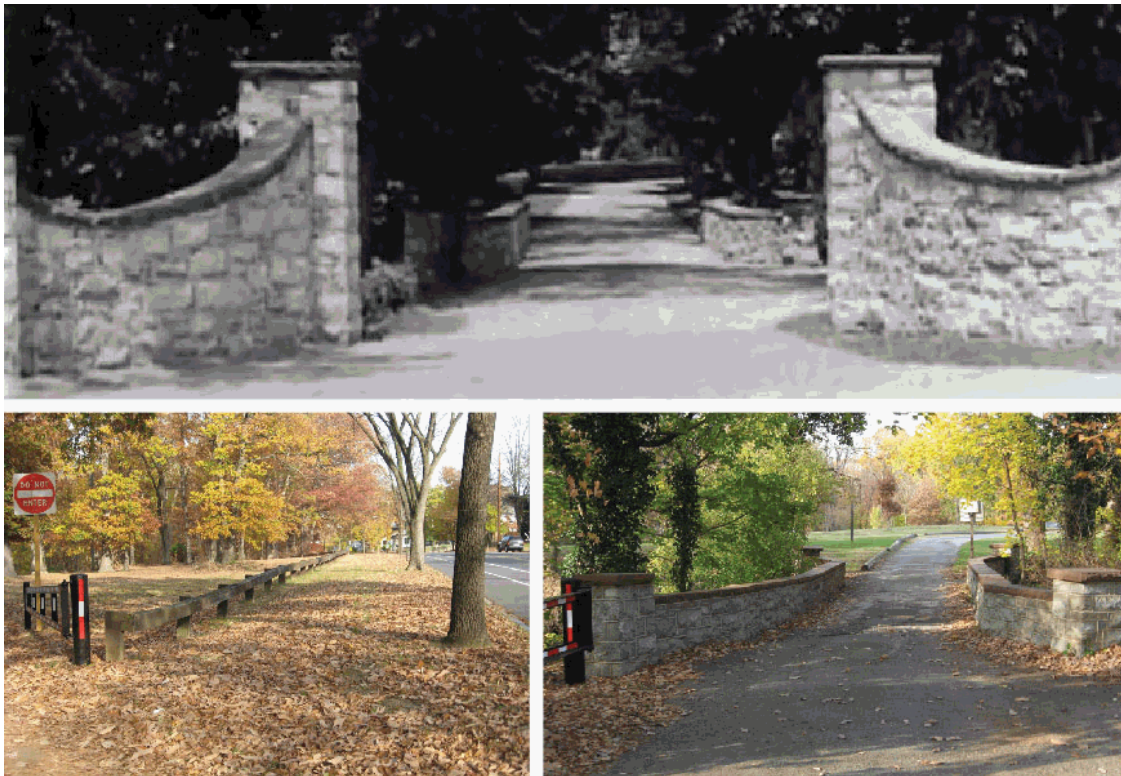
Fort entrance in 1932 (top) & today (bottom). The taller walls from 1932 are no longer extant. The shorter bridge walls (center top; bottom right) were rebuilt in the early 1950s. (Top: Office of Motion Pictures, USDA; Bottom: CLP, 2012)
