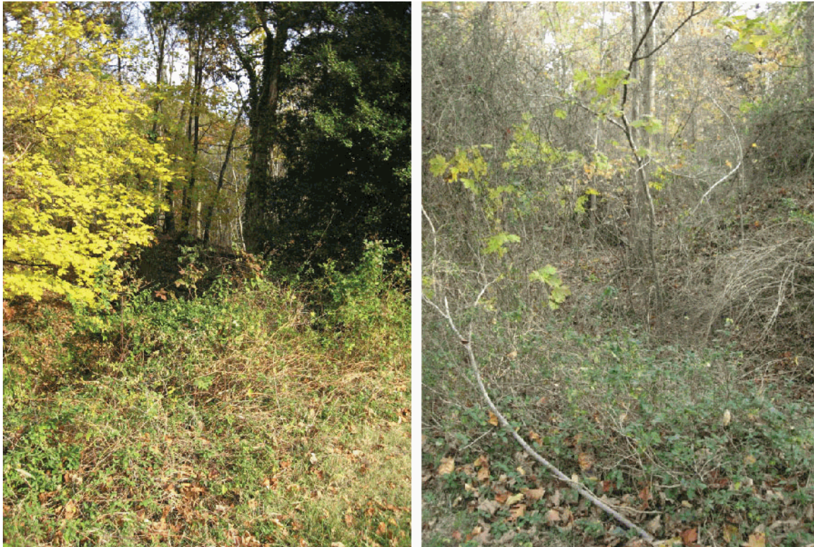
The existing views and vistas from Fort Dupont are obstructed by growth on the earthworks. This disrupts any integrity of views from the fort, which originally looked towards the other forts. (CLP 2012)
