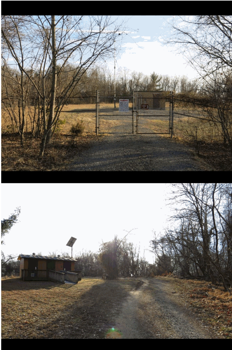
Fig 30 Upper: F.A.A. transmitter Lower: Comfort station and gravel road leading to F.A.A. transmitter (2014 CLP/NCR).
