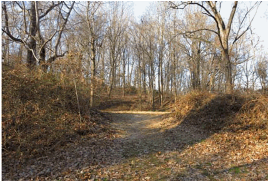
Main Fort, showing portion demolished at unknown date, photo taken by author, December 2014.
