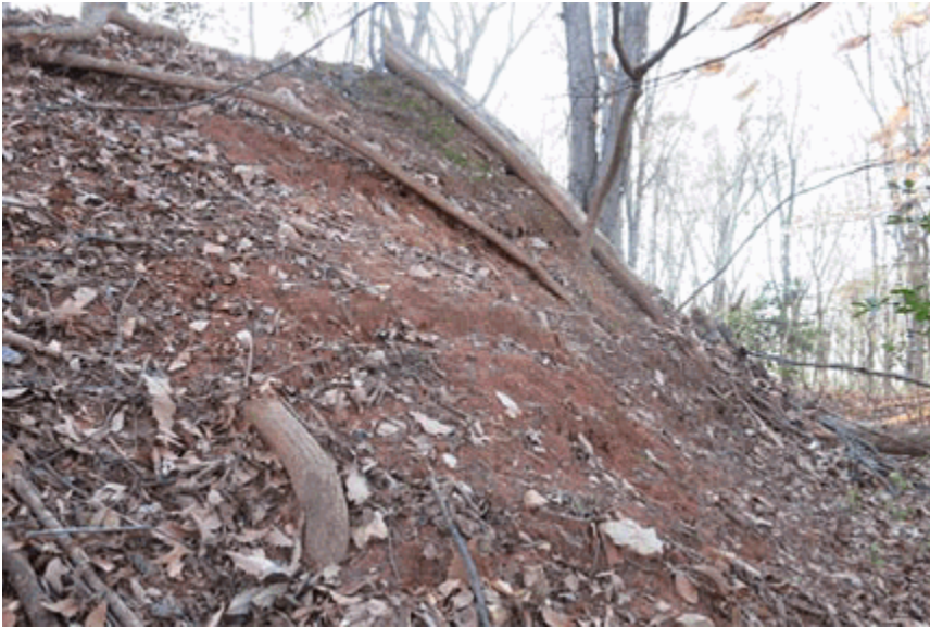
Main Fort, erosion of parapet, photo taken by author, December 2014.
