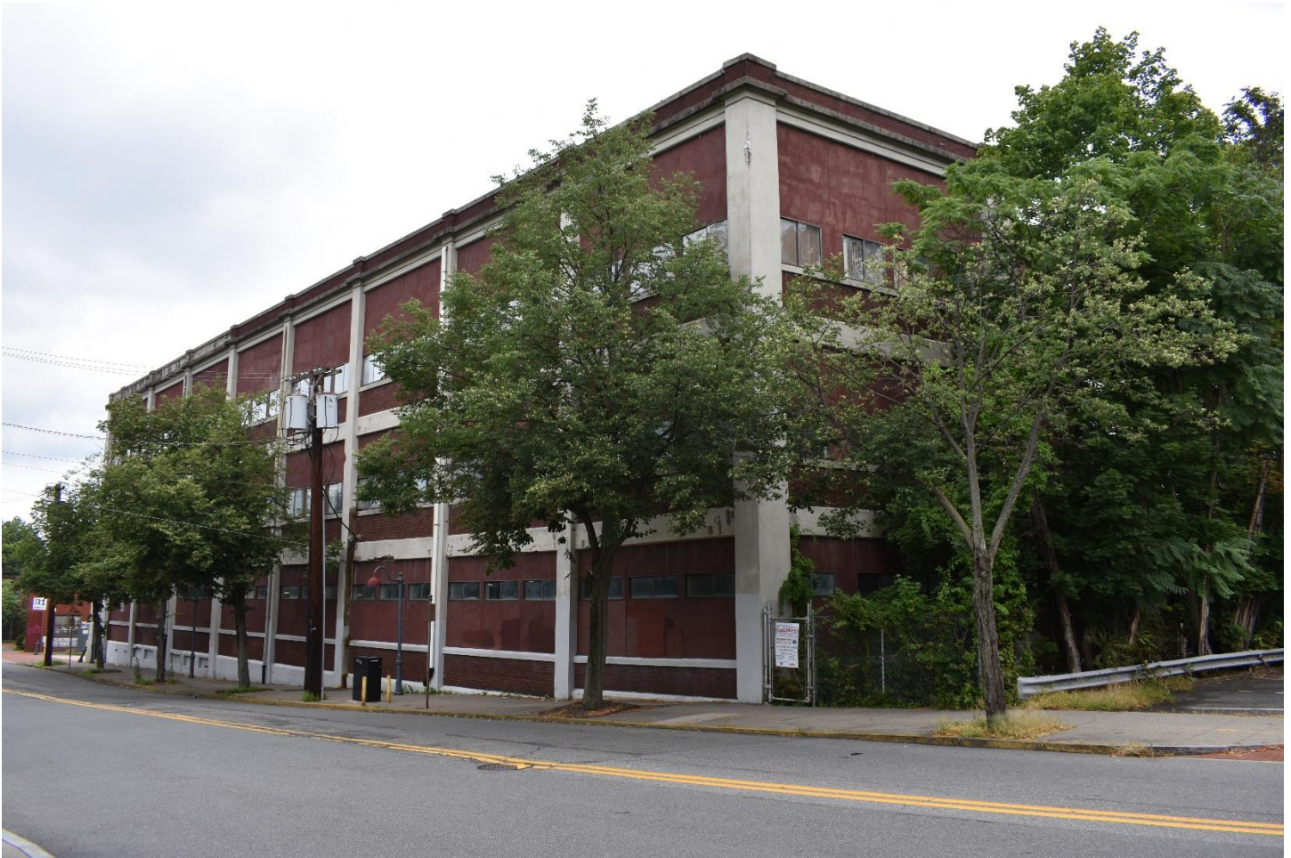
FIGURE 8: Glenro Building, 2017. Photo by the nomination author.
