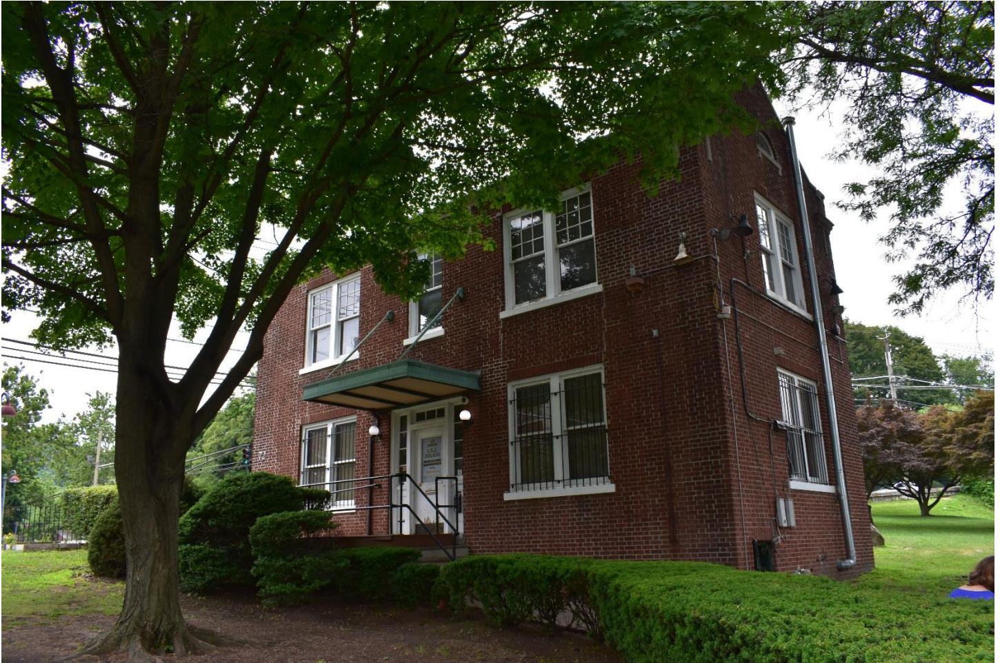
FIGURE 9: S.U.M. Administration Building, 2017. Photo by the nomination author.
