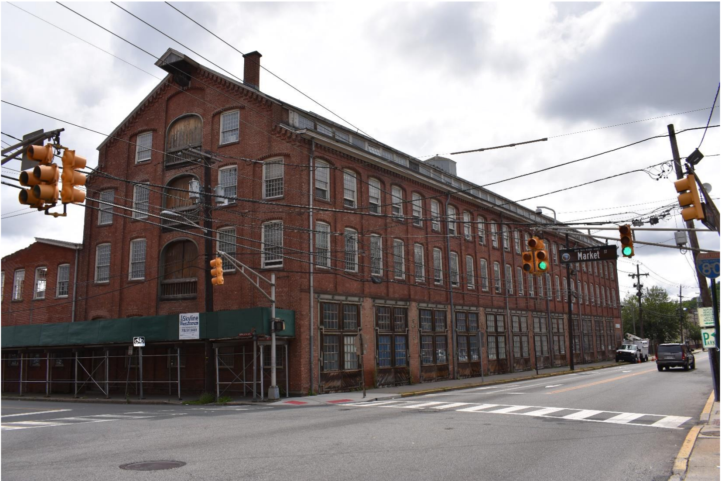
FIGURE 7: Rogers Locomotive Company Erecting Shop, 2017. Photo by the nomination author.
