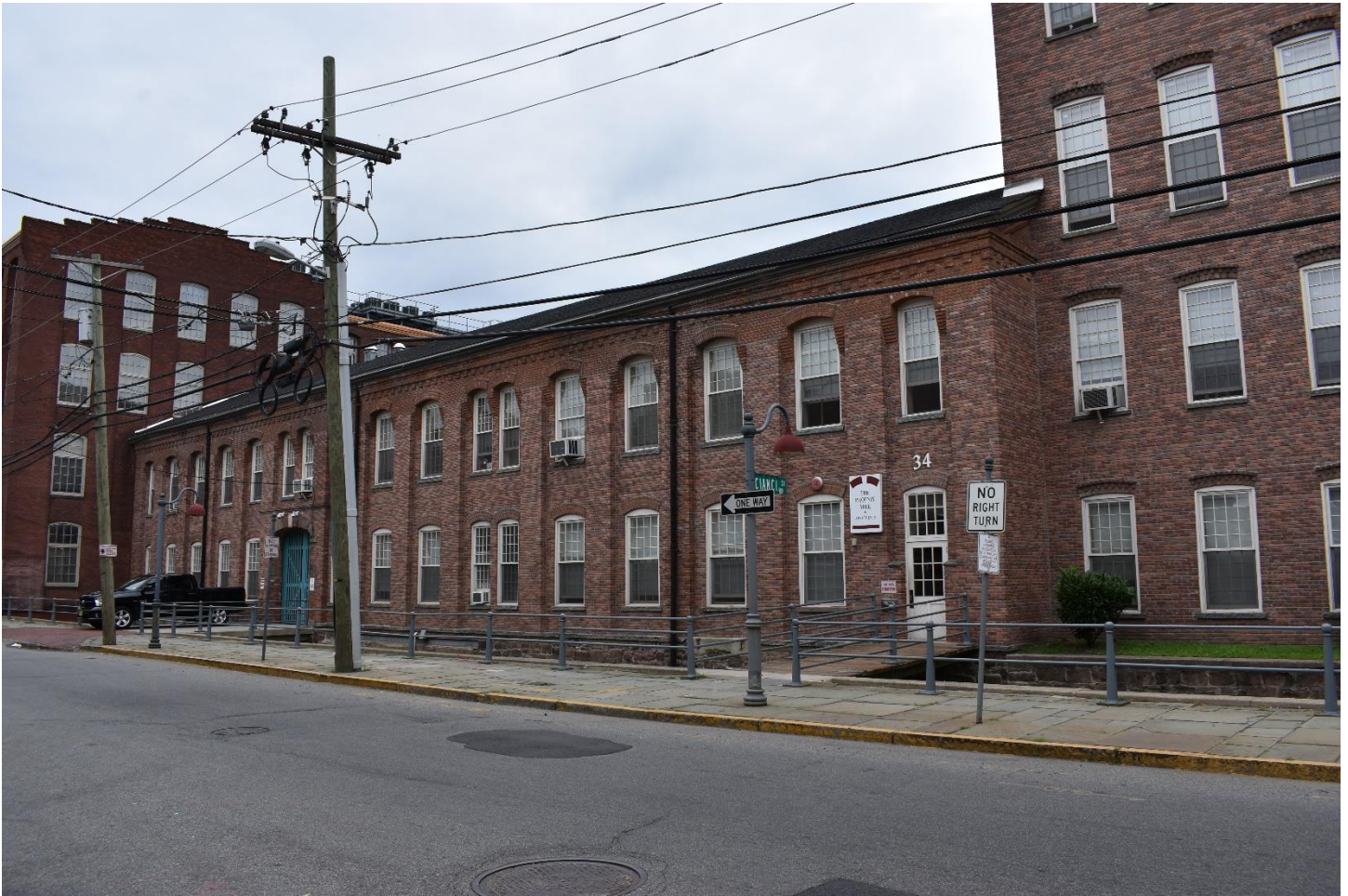
FIGURE 22: Phoenix Mill, 2017. Photo by the nomination author.
