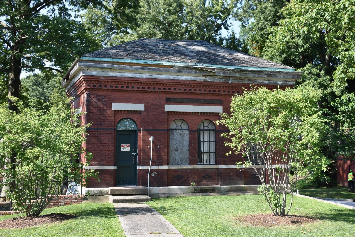
FIGURE 30: Remains of 1876 Steam and Boiler Plant, 2017. Photo by the nomination author.
