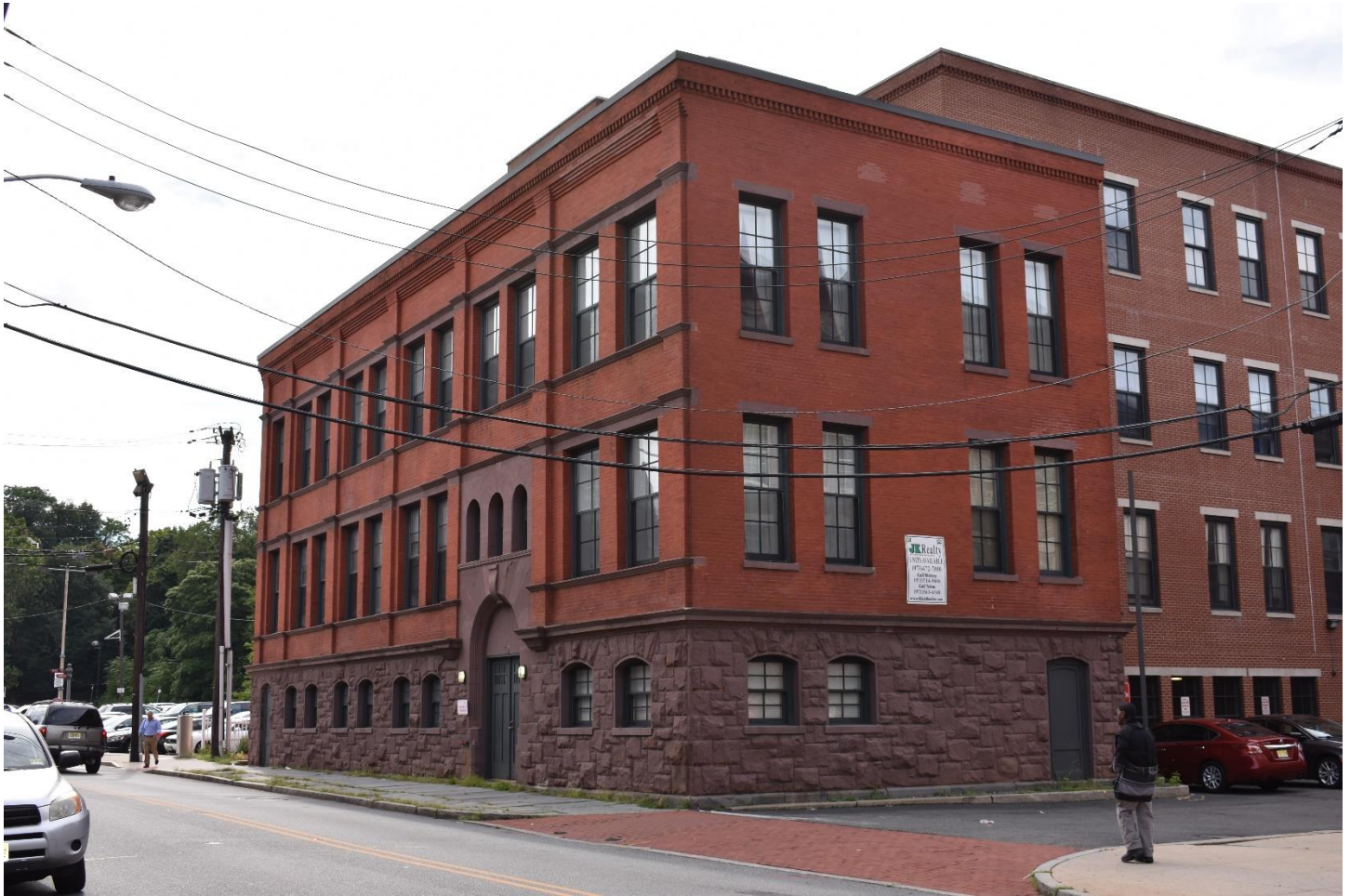
FIGURE 14: Cooke Locomotive Company Office Building, 2017. Photo by the nomination author.
