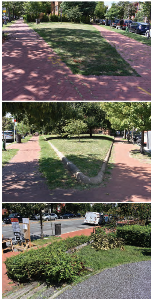
FIGURE 38: The topography within the Maryland Avenue NE cultural landscape varies between reservations graded at the sidewalk (top) and reservations graded at the curb level (middle). Reservation 209 (bottom) has a steeper slope than most of the other reservations; it features a level playing area at the center of the site before sloping down toward Maryland Avenue NE. (Photographs by the CLI author)
