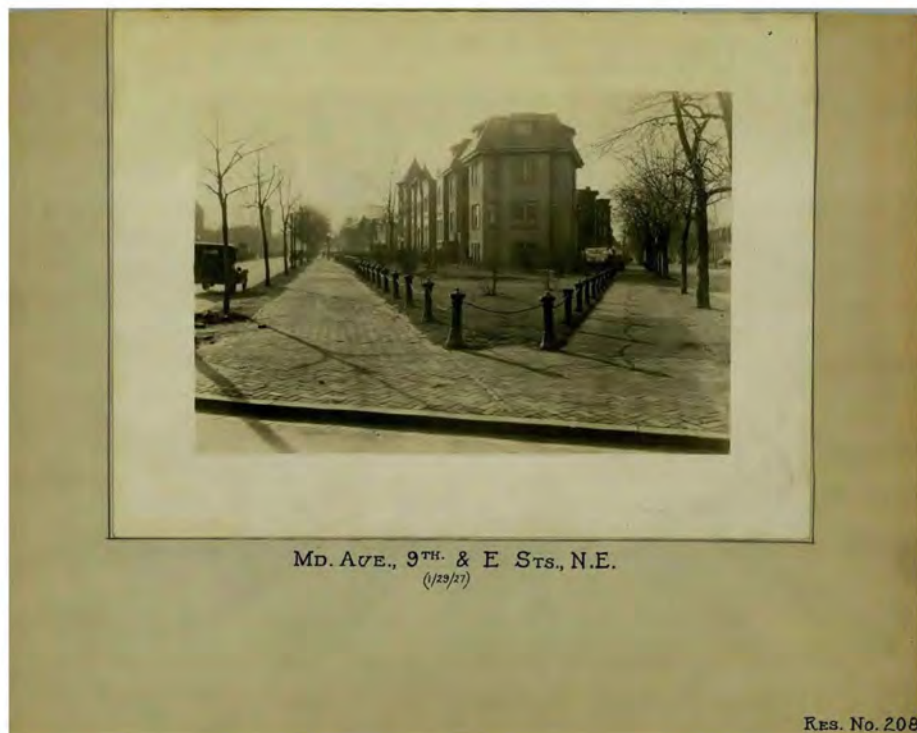
FIGURE 17: Reservation 208, as seen in 1927 survey conducted by the Office of Public Buildings and Public Parks. (Reservation 208, Reservation Files, National Capital Area)
