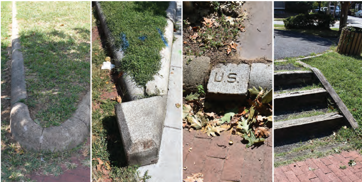
FIGURE 50: The cultural landscape retains several significant small-scale features, including intact curbing from the OPBG era (left and center-left), “U.S.” marker stones installed by OPBG (center-right), and rail-tie steps installed as part of the Beautification Program’s projects (right). (Photographs by the CLI author)
