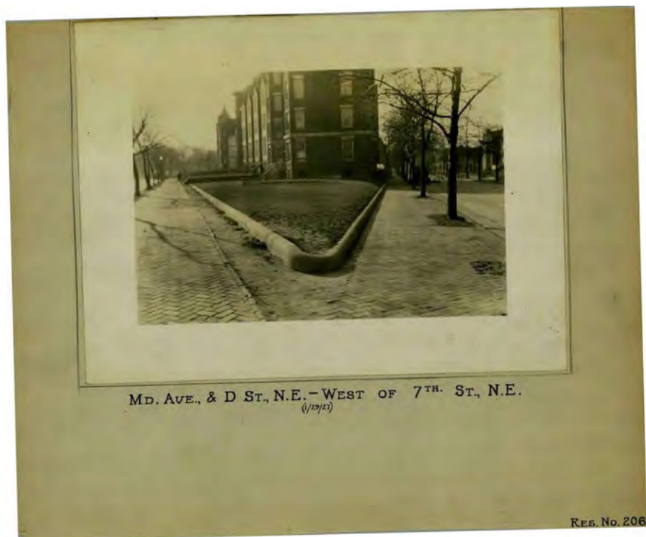
FIGURE 15: Reservation 206, as seen in 1927 survey conducted by the Office of Public Buildings and Public Parks. (Reservation 206, Reservation Files, National Capital Area)
