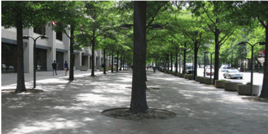
Current Condition of Pennsylvania Avenue Street Trees. Many of the street trees have overgrown their surrounding custom tree grates, and such constriction has negatively impacted the trees' health. In eight cases, unhealthy trees have been removed and onl
