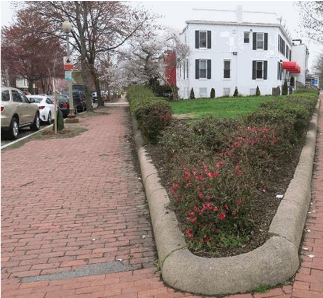
Figure 27: Quarter-round curbing at Reservation 052
