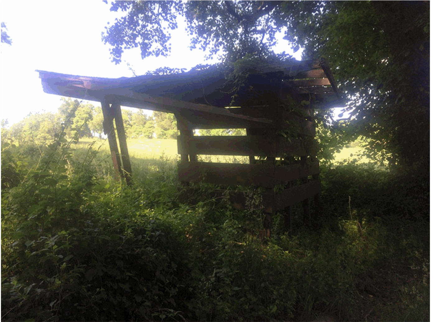
Shelter dating to second period of significance, dismantled in fall 2016.
