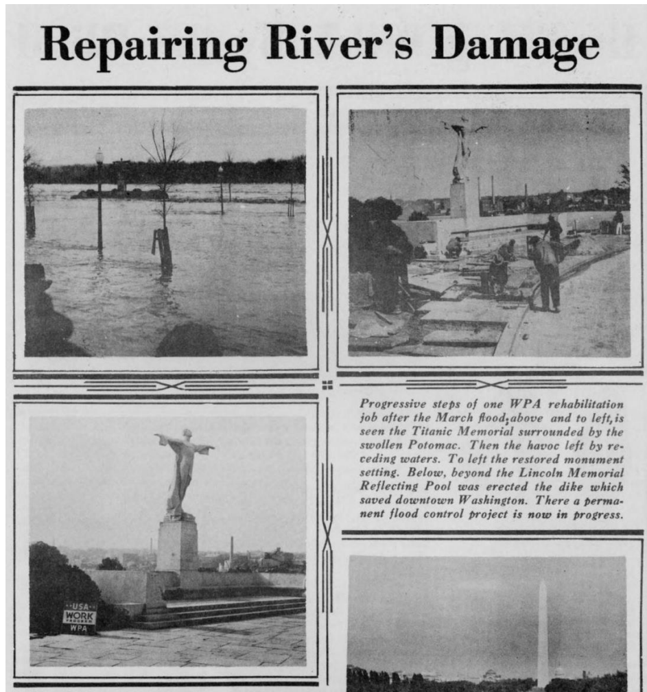
FIGURE 32: In 1936, WPA workers rehabilitated the Titanic Memorial sculpture at its site along the Rock Creek and Potomac Parkways after a flood caused significant damage to the sculpture. (“Repairing River’s Damage,” Work: A Journal of Progress , Vol, 1, No.1, 1936: 13)
