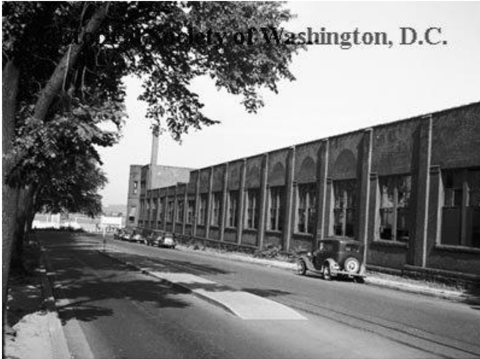
FIGURE 34: View to the northwest of the Capital Transit Company 7th Streetcar barn on the north side of P Street SW. Prior to redevelopment, the cultural landscape featured a raised trolley platform and a row of elm trees along P Street SW. (August 6, 1950, WY 3431.49, John P. Wymer photograph collection, Historical Society of Washington, DC)
