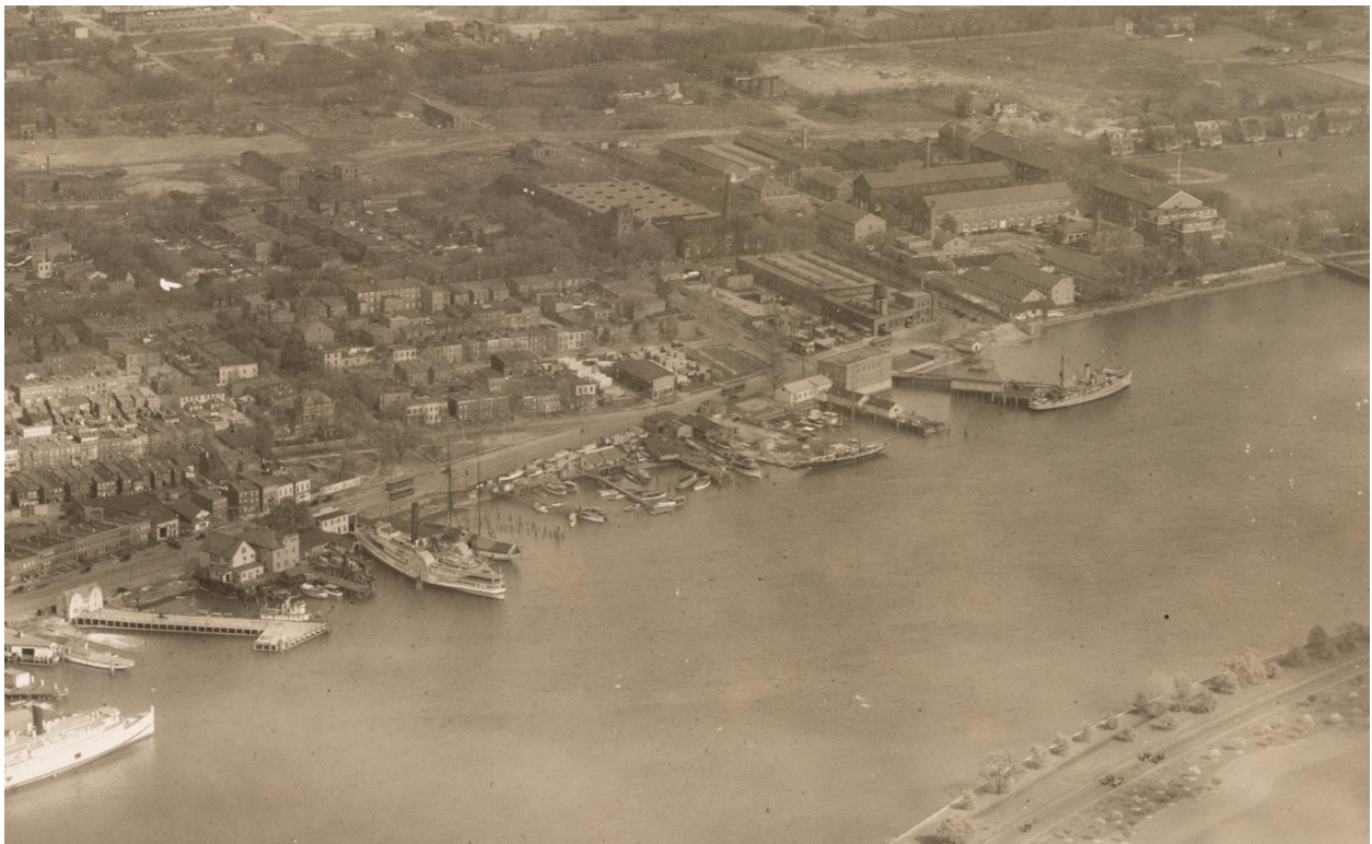
FIGURE 30: This 1925 aerial photograph shows the southwest waterfront and the cultural landscape. By this time, the cultural landscape was in use as an active transportation corridor. Conditions remained largely consistent with previous eras. (Excerpt from Record Group 18-AA, "Airscares" of American and Foreign Areas, Box 150, Folder 24, National Archives and Records Administration)
