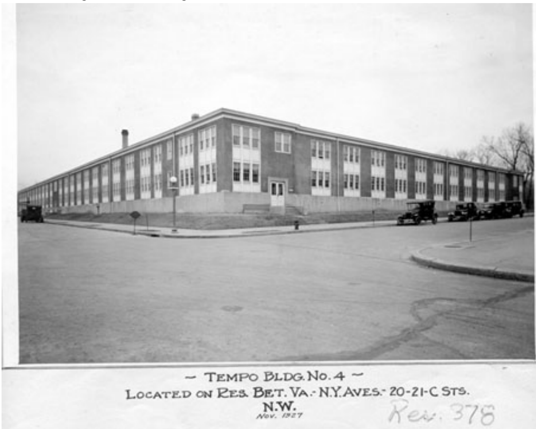
Temporary office building erected on Reservation 105 (Edward J. Kelly Park)/378 (Federal Reserve Annex) during World War I. OPBPP Survey Photo, 1927. NPS Land Files.
